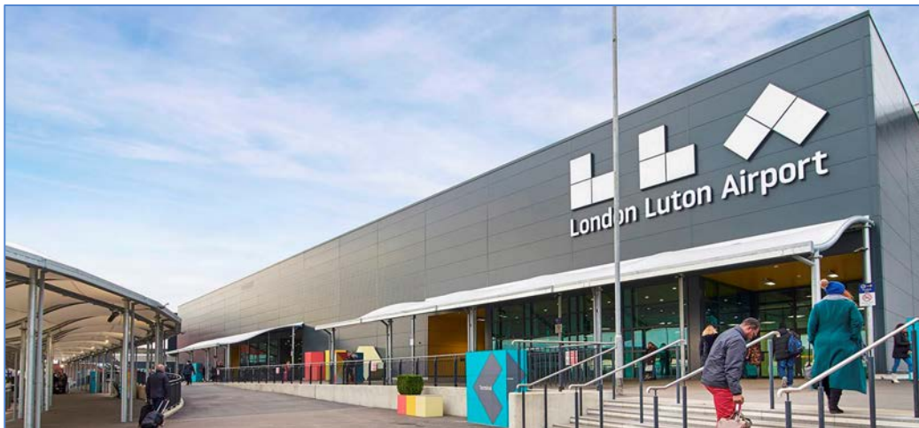
Figure 20 - London's Luton Airport arrival terminal
